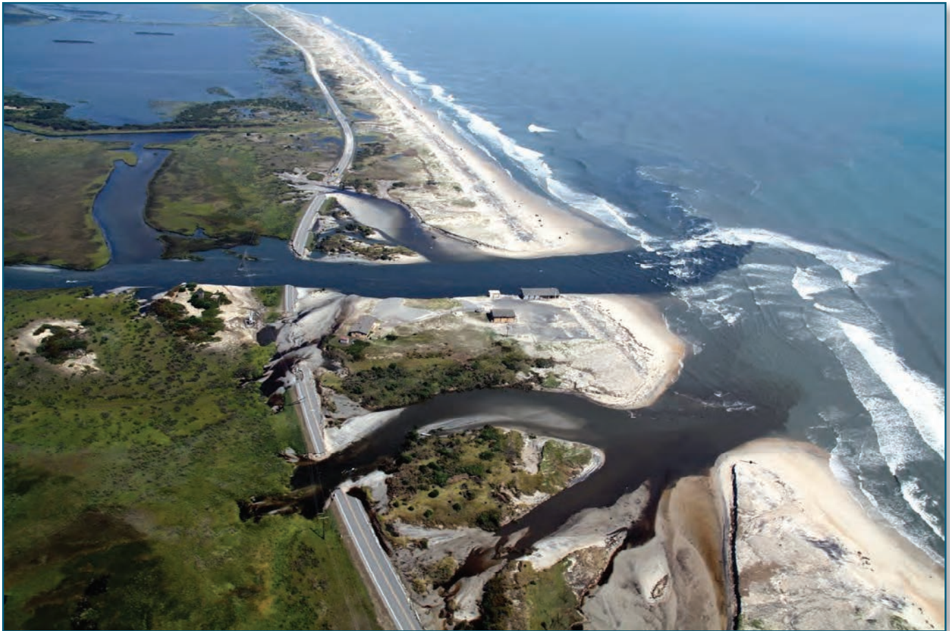
Figure 5. Storm damage and saltwater inundation resulting from Hurricane Irene along the coast of North Carolina, 2011. 8 In addition to the property damage and threats to coastal residents, the frequency and intensity of coastal storms can also influence coastal wetland types and distribution through erosion, deposition of sediments or by increasing salinity.
